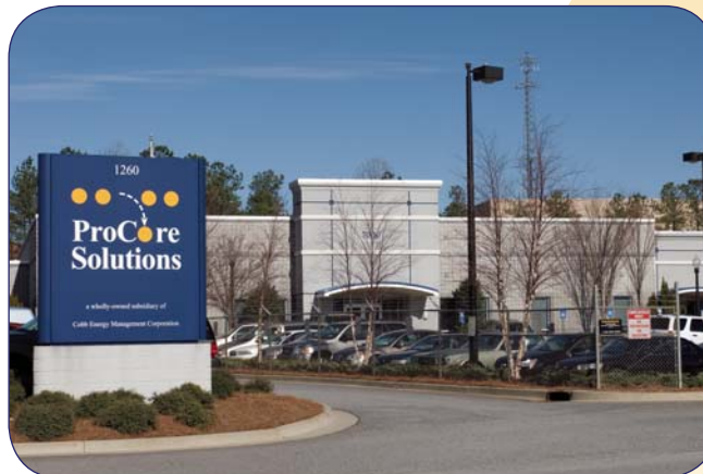
ProCore's Marietta, Ga., facility.
